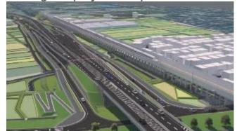
The Yasu-Ritto Bypass is a 4.7km long road that was put into operation in 1982 with the aim of easing traffic congestion on National Route 8 between Yasu City and Ritto City. The construction involves constructing the superstructure of the main line and the on and off ramps.
